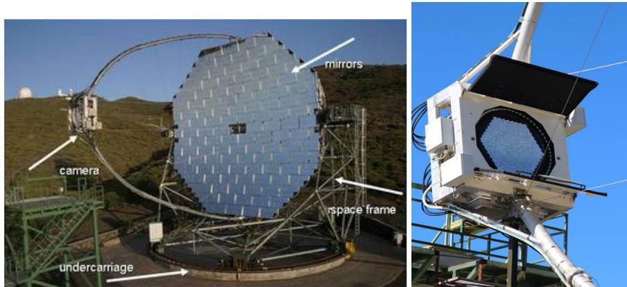
(a) Structure of the telescope. (Image taken from the MAGIC Telescopes webpage <sup>2</sup>)
